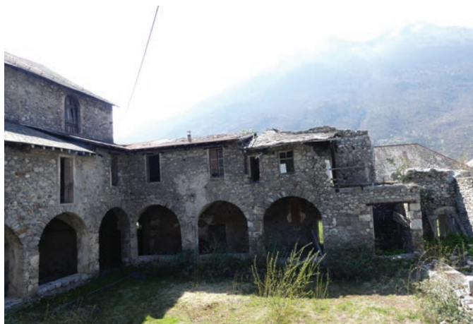
ph15) Cloître aile Ouest façade Est 2022 (D. Perron)
