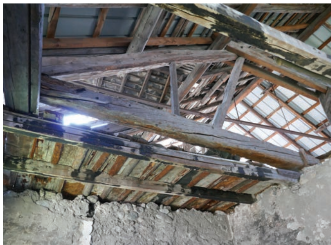
ph58) charpente salle capitulaire 2022 (B. Chambre)
