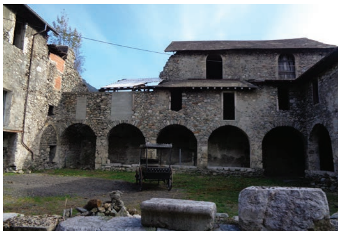
ph26) Cloître aile Sud façade Nord 2019 (D. Perron)
