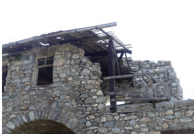
ph20) Cloître aile Ouest façade Est 2022 (D. Perron)
