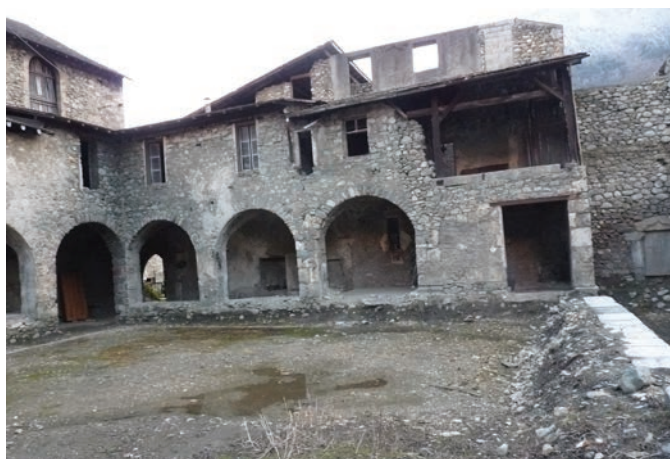
ph13) Cloître aile Ouest façade Est 2010 (D. Perron)
