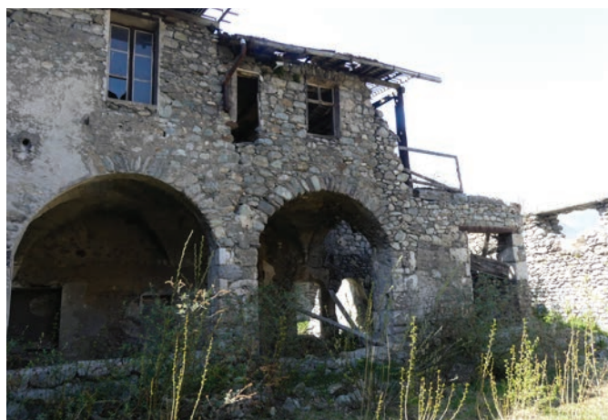
ph18) Cloître aile Ouest façade Est 2022 (D. Perron)
