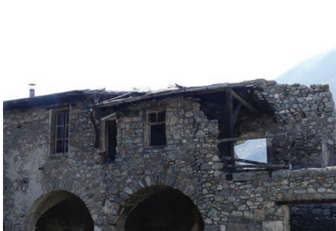
ph17) Cloître aile Ouest façade Est 2022 (D. Perron)
