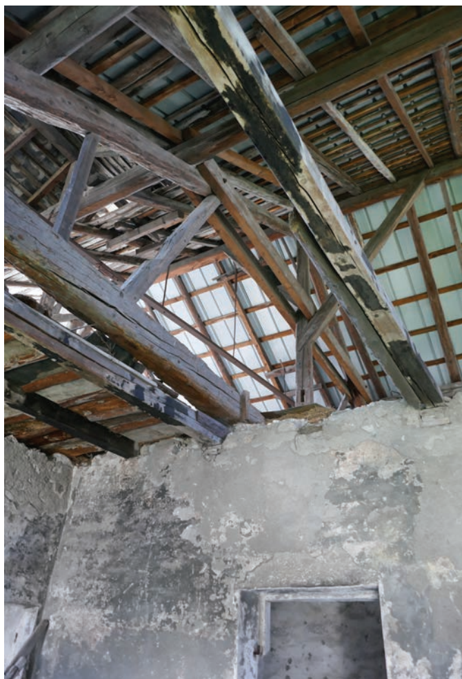
ph56) charpente salle capitulaire 2022 (B. Chambre)
