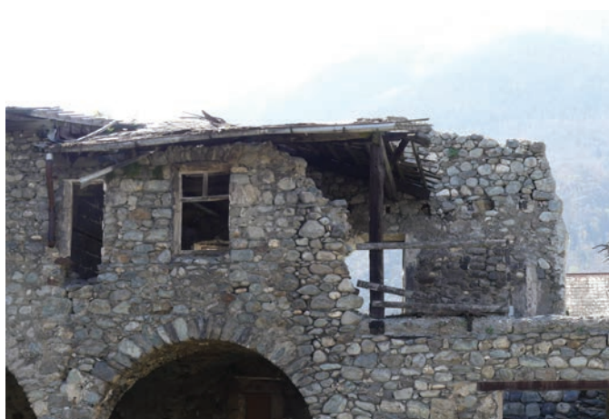
ph19) Cloître aile Ouest façade Est 2022 (D. Perron)
