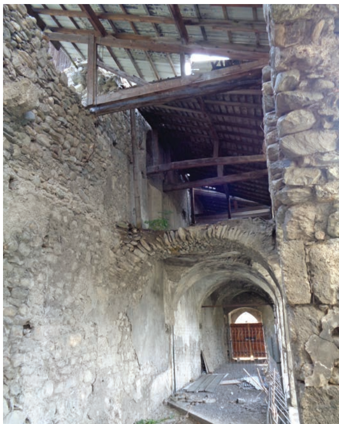
ph31) Cloître aile Sud façade Nord 2019 (D. Perron)
