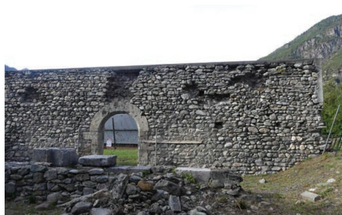
ph7) Mur Nord façade Sud 2019 (D. Perron)
