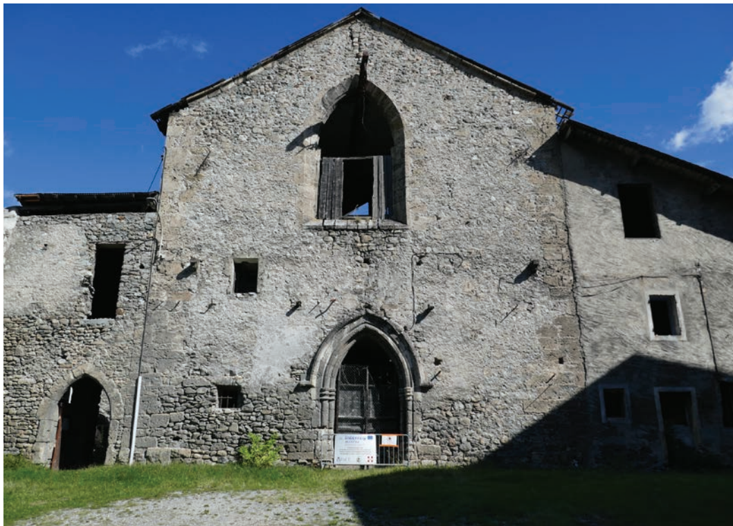
Ph71) Eglise façade Ouest 2021 (D. Perron)
